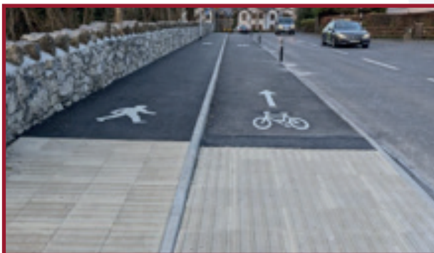
New Cycle Path completed at Boys School on Maree Road
